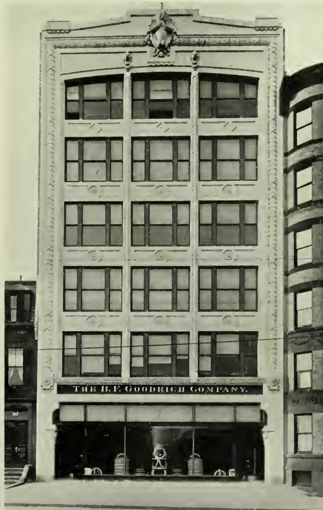
STORE BUILDING, BOYLSTON STREET, BOSTON. Front of light cream matt glazed terra cotta furnished by the Atlantic Terra Cotta Company. Kendall & Taylor, Architects.
